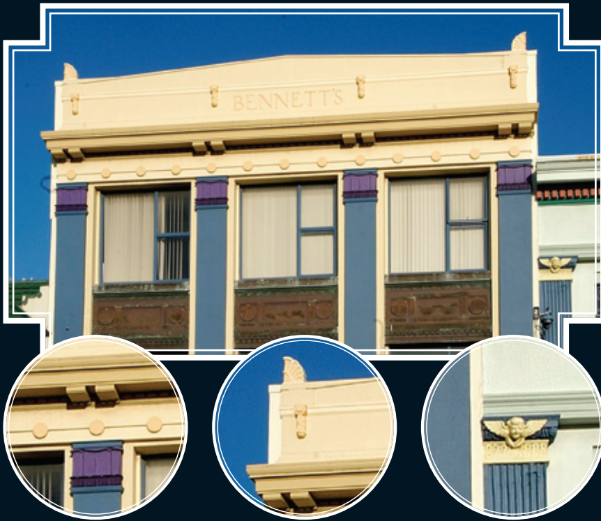
Bennett's Building: Side walls and edges of front wall: Resene Dutch White, front wall: Resene Chamois, eyebrow above windows: Resene Putty, palmettes and bands: Resene Cherokee and Resene Casablanca, columns: Resene Astronaut, Resene Blackcurrant and Resene Scarlet Gum, aluminium windows and veranda hangers: Resene Astronaut.
