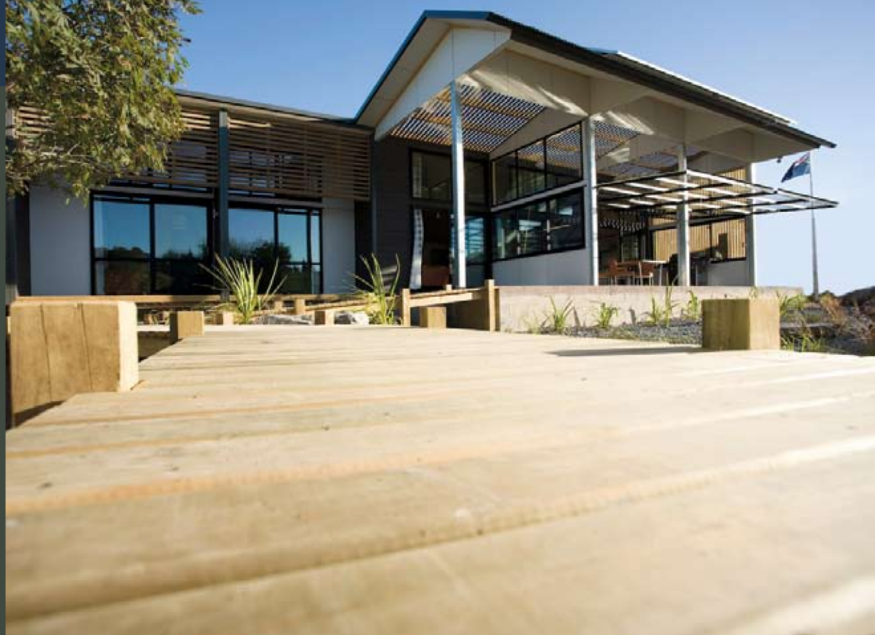
Right Large double-glazed windows on the northern side of the house welcome in the sun's warming rays.
